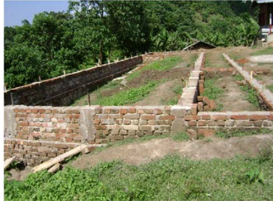
Incomplete Construction of girl dormitory
