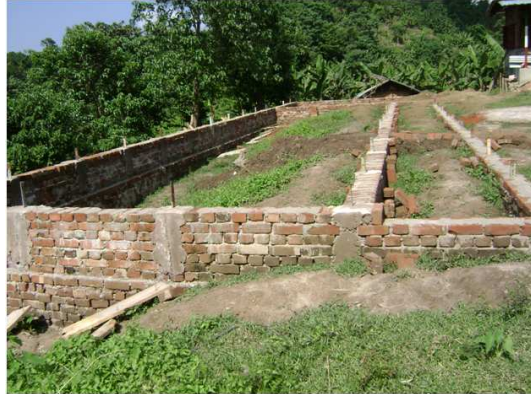
Incomplete Construction of girl dormitory
